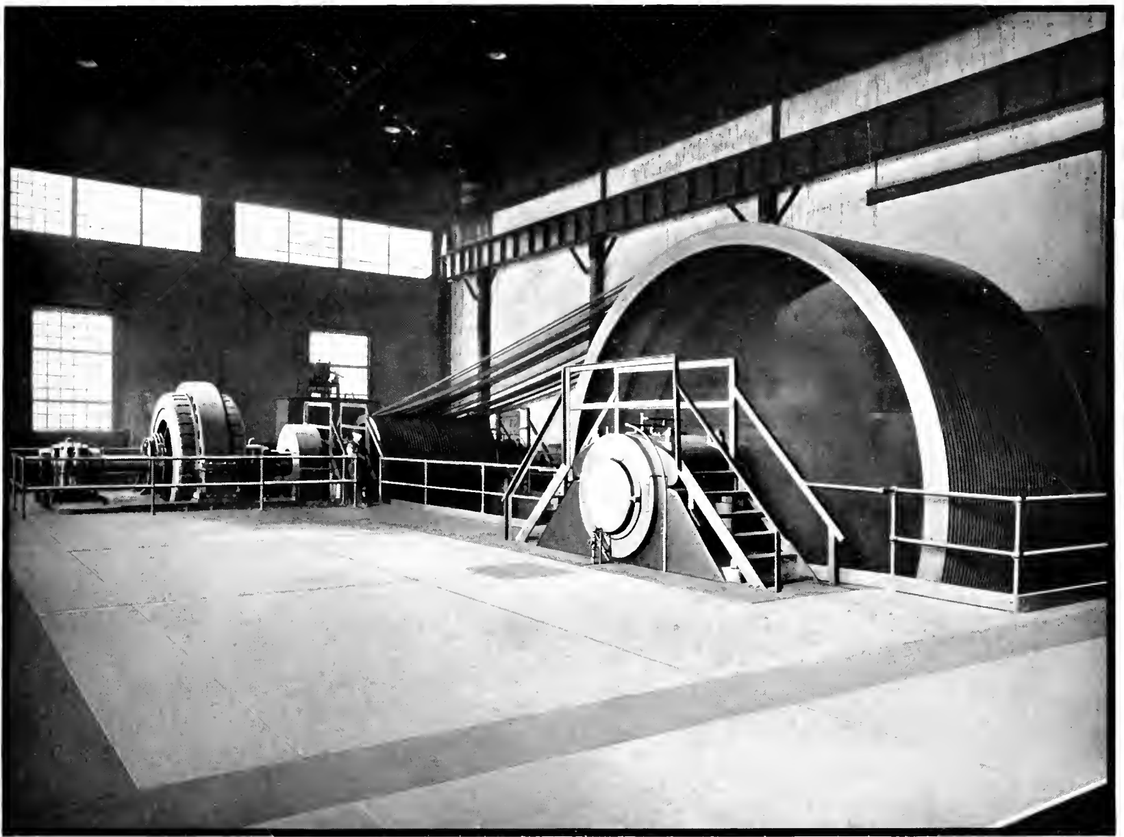
Mesta Rope Drive Installed at The Inland Steel Company
